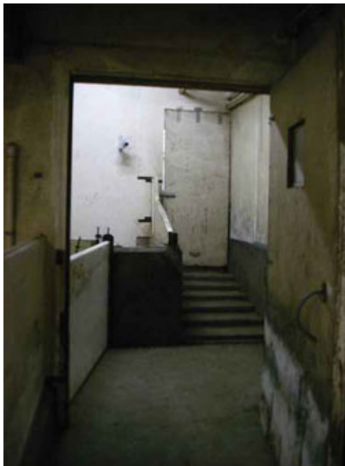
Figure 2. Well lit load-out with concrete steps (30-cm treads). Although this load-out involves some corners, the transitions are smooth and well-lit and the alley is wide enough for multiple pigs to pass
